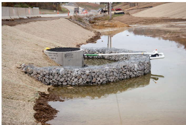
Fig. 4.14. Faircloth skimmer at Sediment Basin 1.
