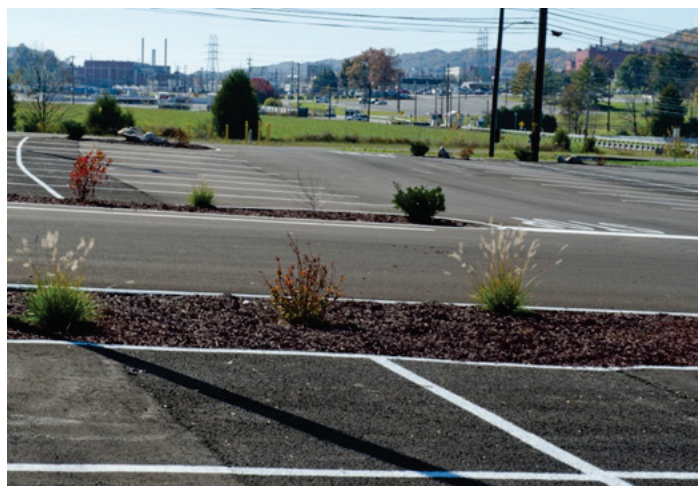
Fig. 4.15. Permeable pavement and native planting contributes to compliance with EISA 438 requirements. [Source: Kathy Fahey, Y-12 Photography.]
